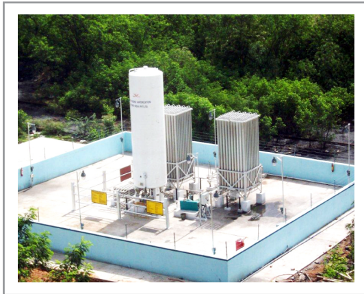
CRYOGENIC TURNKEY INSTALLATION, LP & HP LOX TURNKEY INSTALLATION
