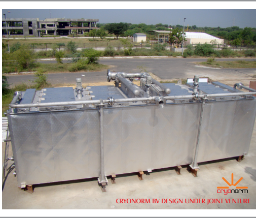
STEAM HEATED WATER BATH VAPORIZER
