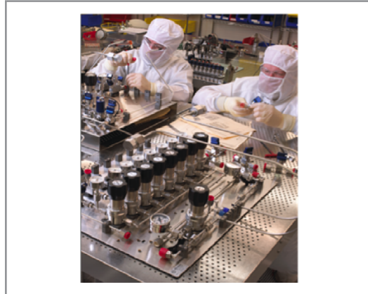
CLASS 100 CLEAN ROOM FOR PANEL FABRICATION
