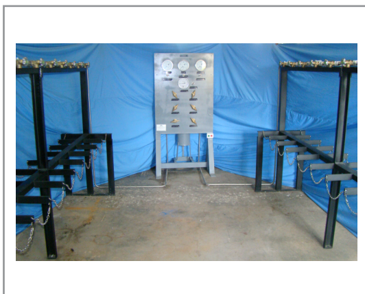
GROUND MOUNTED CYLINDER FILLING MANIFOLD & CONTROL PANEL
