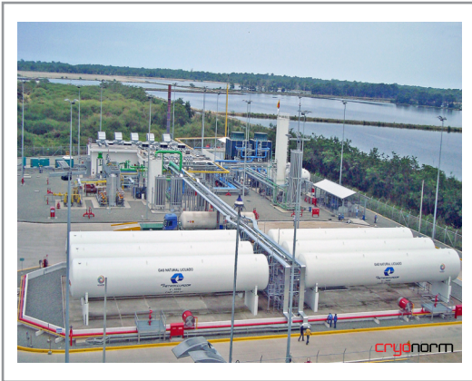
200 MT LIQUEFACTION PLANT AS EPC PROJECT
