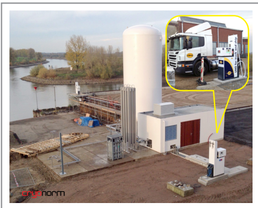
LNG STORAGE & DISPENSING FOR TRUCKS & SHIPS
