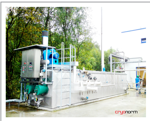
GAS FIRED VAPORIZER
