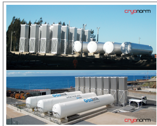
25,000 NM 3 /HR. @ 78 BARG PIPE LINE INJECTION 2 BANKS OF 10 PCS PARALLEL WORKING AMBIENT VAPORIZER
