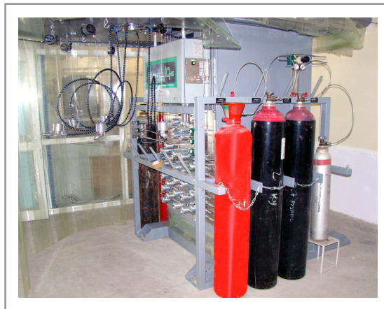
'RECIPE' BASED FULLY AUTOMATED TOUCH SCREEN OPERATED CALIBRATION GAS BLEND STATION
