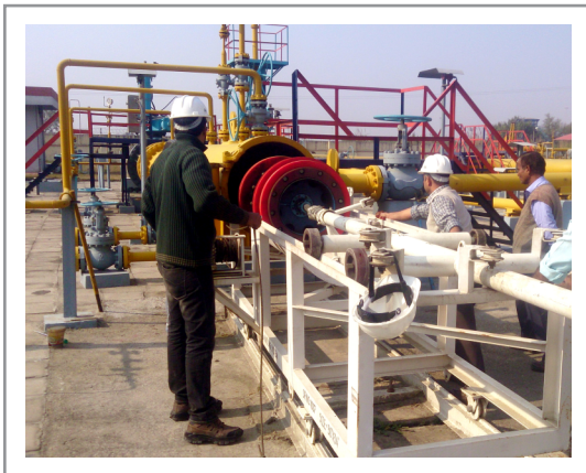
PIGGING PROJECT & PIG LAUNCHING STATION
