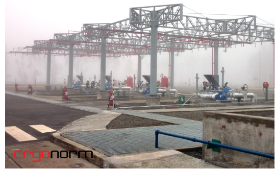
4 BAY SIMULTANEOUS TANKER LOADING TERMINAL AT PORT
