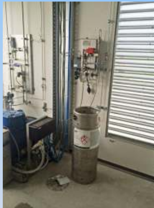
High pressure Odorizer system
