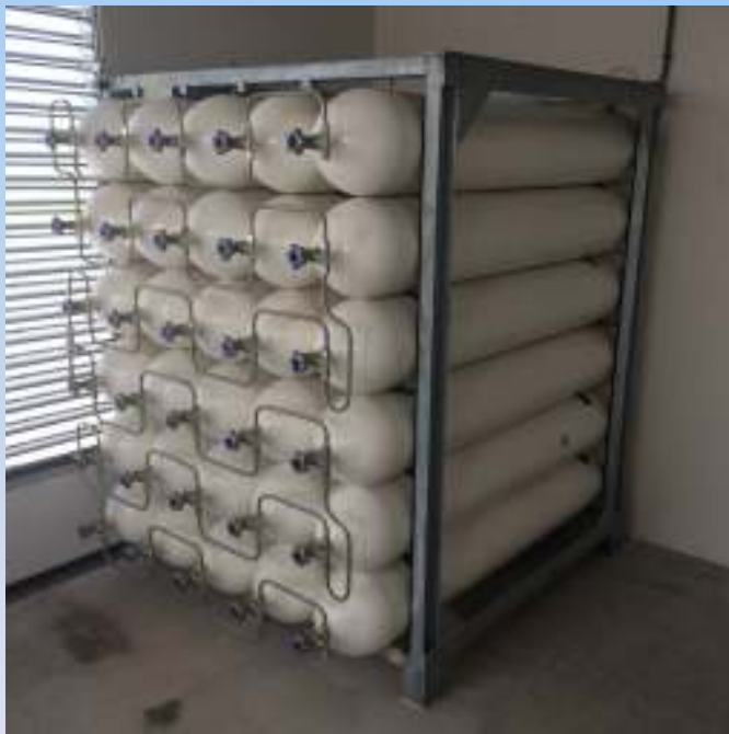
500 Nm 3 @ 200 barg Bottle rack capacity
